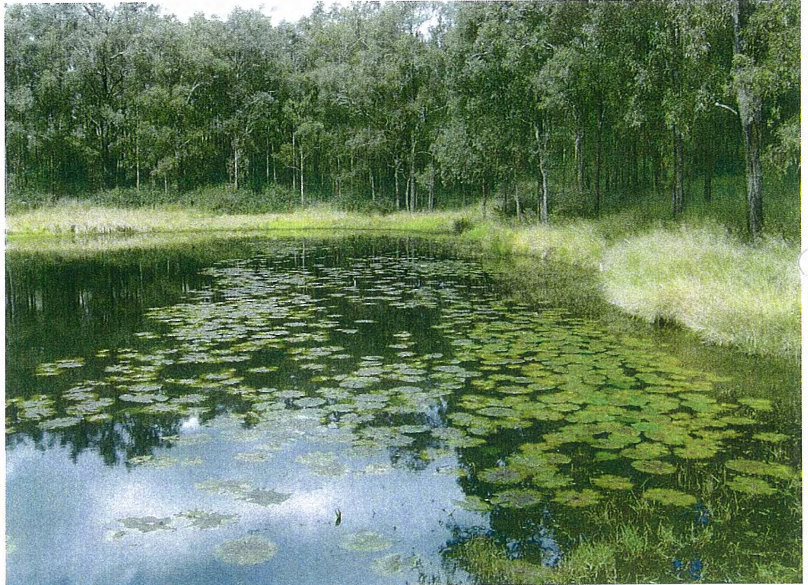
Plate 7: View looking south from northern side of Dam 3
