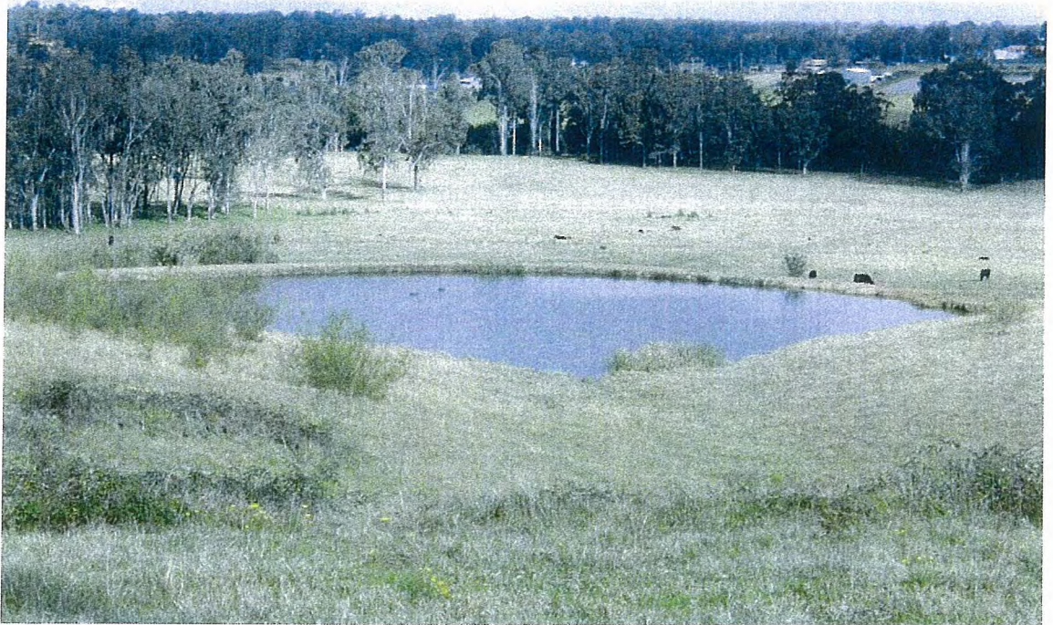
Plate 8: View looking at Dam 5 from the north-west
